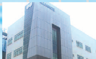
TERASAKI CIRCUIT BREAKERS (S) PTE. LTD. (Singapore)
